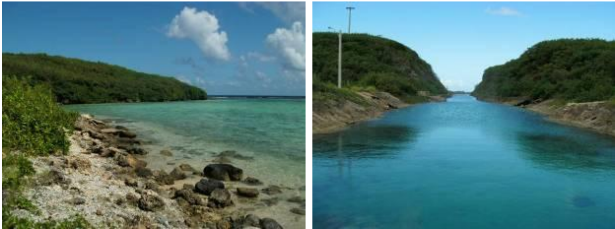
Left: View from Route 11 to northeast. Right: Cooling water canal (Approximately 5 ac (2 ha) with rip rap lining the sides. This canal connects the power plant near the Commercial Port along Route 11 to Piti Bay and the Philippine Sea.
